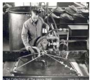
In the Collections of The Henry Ford Soybean Car assembly image showing production of plastic panels.
