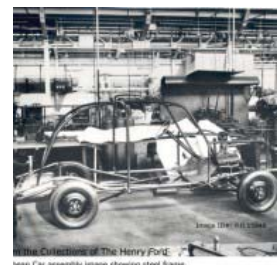
In the Collections of The Henry Ford Soybean Car assembly image showing steel frame.
