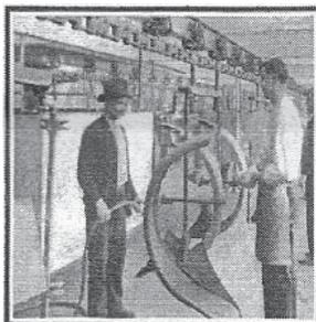
Left: Inspecting Bonderized fenders after they have passed through the process.
